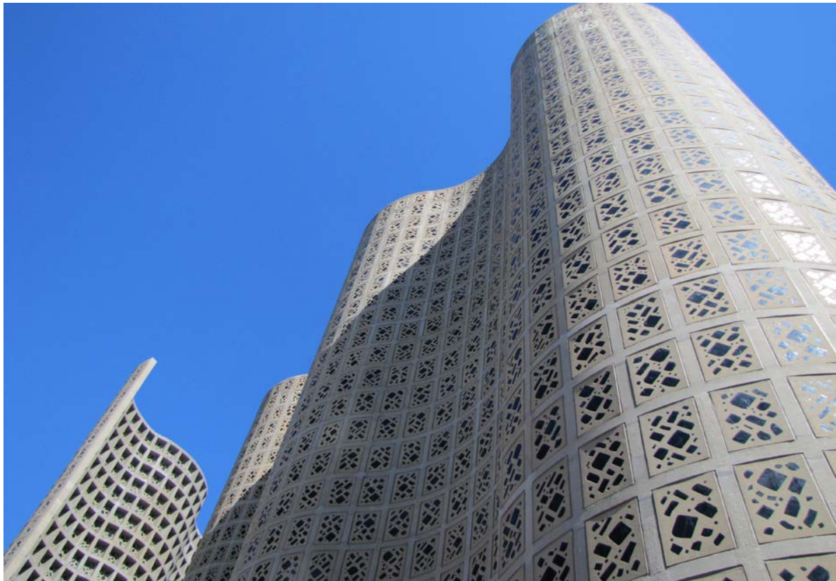
Figure 1. Great Hall façade. The freestanding wall at the left of the image overlaps the serpentine plan to create the original building entrance.
