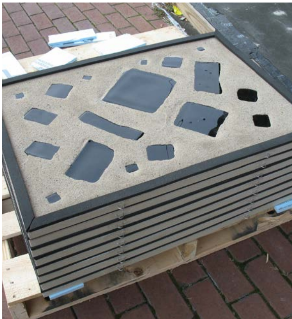
Figure 6. Epoxy replacement panels prepared for installation. The sand broadcast onto the surface of the epoxy creates a finish similar to the original concrete matrix.
