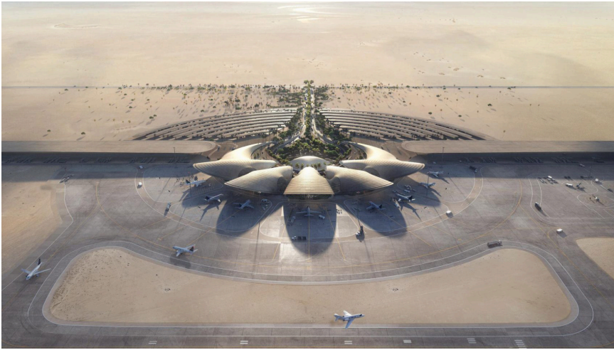
Image 8.10. Rendering showing Red Sea International Airport, designed by Foster Partners. Courtesy of TRSC / Foster Partners.
